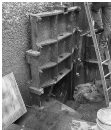
Existing sluice gate
