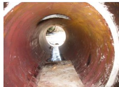
New sluice pipe liner gouted in place
