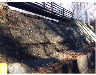
As can be seen in this photo, the face of the main spillway is spalling and deteriorating. An area just west of the main spillway looks the same. This project will require chipping away approximately 6" of deteriorating concrete face, installing pins grouted into the remaining sound concrete dam, installing a grid of epoxy coated steel reinforcing bars, and forming and pouring a new concrete face to the main spillway and adjacent area. Approximately 620 square feet of
